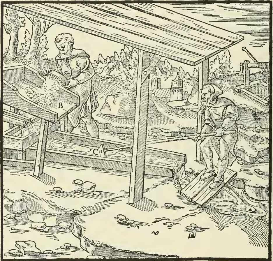
A—TROUGH. B—PLATFORM. C—WOODEN SCRUBBER.
